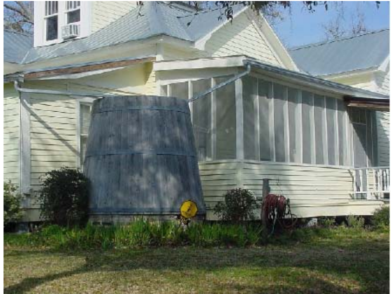
Figure 2 Above-ground cistern located at the corner of a house near existing downspouts.
