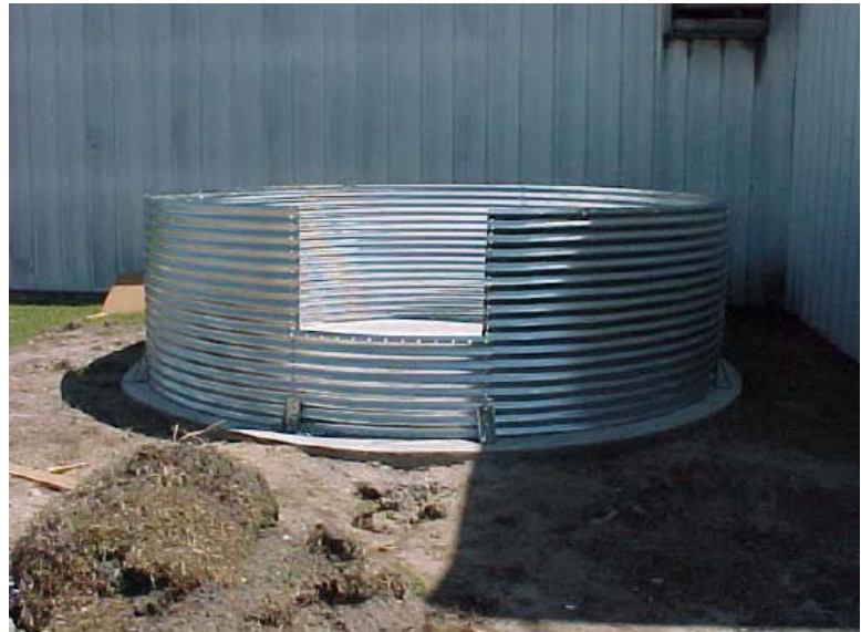
Figure 3 Metal cistern being constructed.
